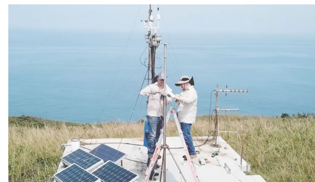
Equipment installation in outstation
