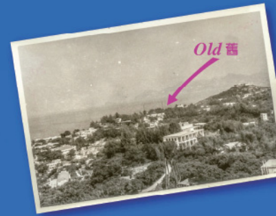
一九五三年建成的舊長洲航空氣象站。 The old Cheung Chau Aeronautical Meteorological Station set up in 1953.
