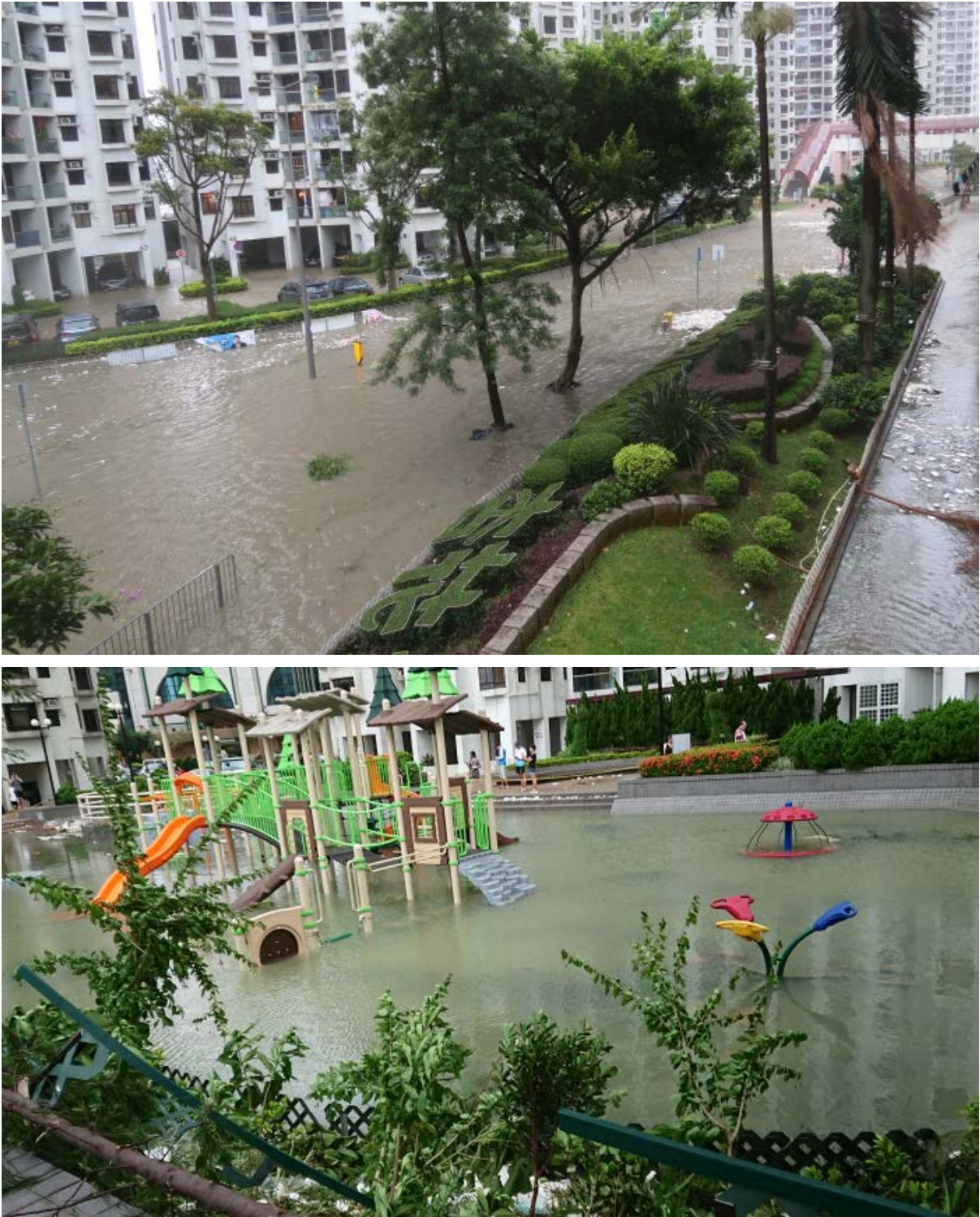
圖 3.3.15a 杏花邨一帶嚴重水浸，海水湧入邨內。(圖片鳴謝: Steve Lee 和岑富祥) Figure 3.3.15a Heng Fa Chuen was seriously flooded with sea water rushing into the estate. (Photos courtesy of Steve Lee and F. C. Sham)
