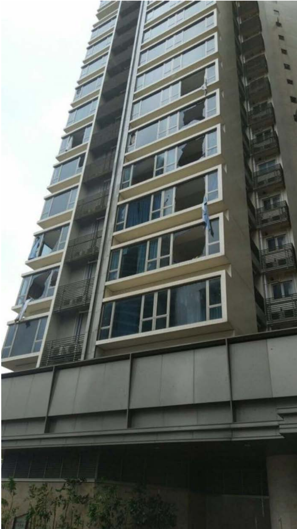
圖 3.3.21 澳門有住宅大廈的窗戶玻璃爆裂。(圖片鳴謝: 方志剛) Figure 3.3.21 Window panes of residential buildings in Macao were broken. (Photo courtesy of Clarence Fong)
