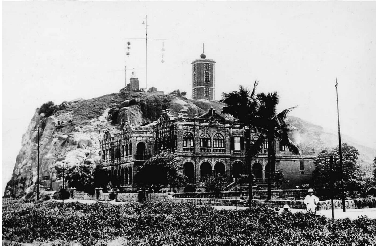
Figure 12. Display of the China Seas Storm Signal Code on Signal Hill in the 1920s. The symbol at the mast head showed the time the warning was issued. The symbols displayed under the yard-arms represented the position of the centre of the storm (left) and the direction of movement and certain characteristics of the storm (right) (courtesy of Mr. Shun Chi-ming).
