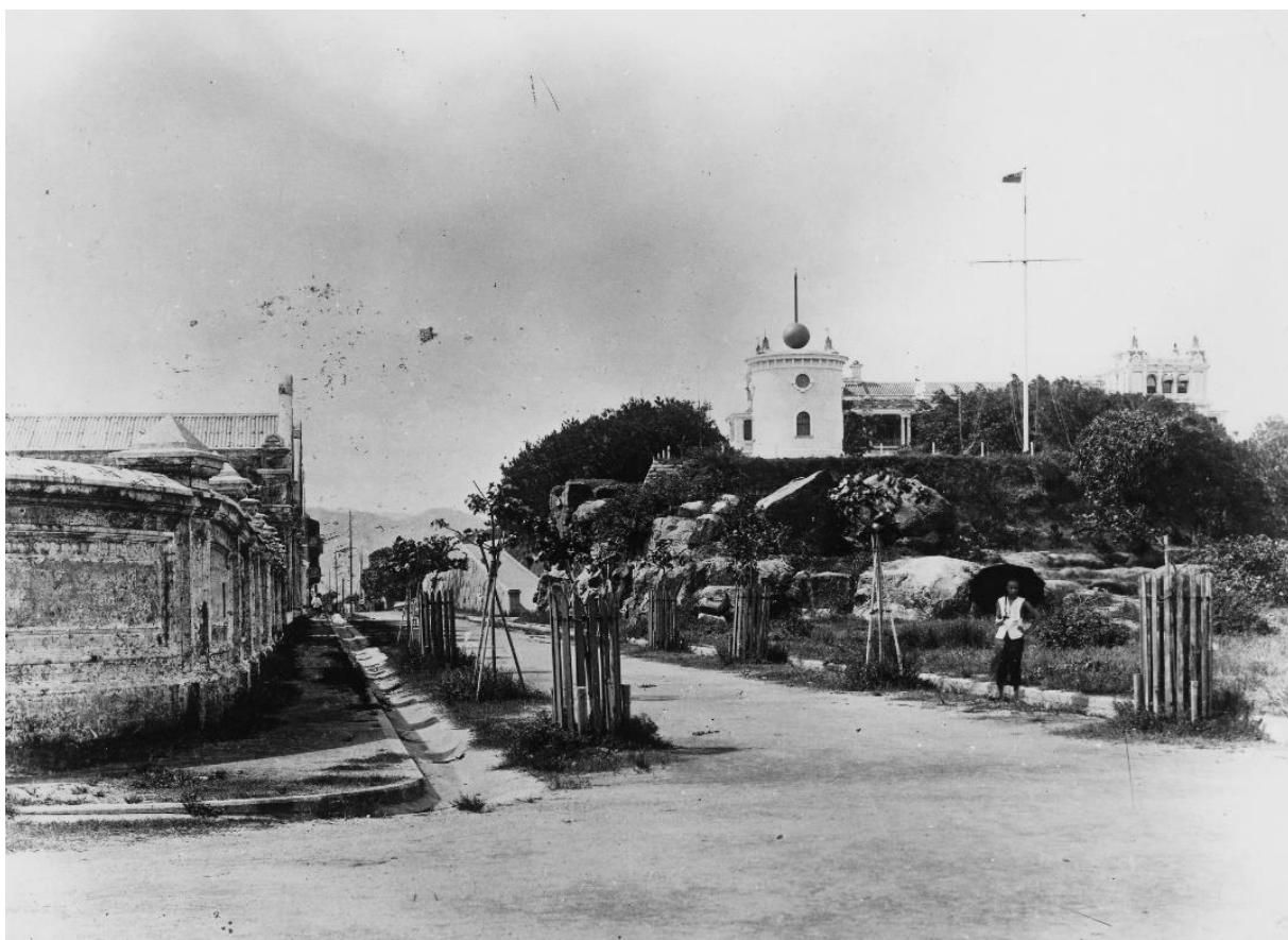
Figure 5. The Time Ball at Tsim Sha Tsui Police Barracks (Water Police Station). Meteorological signals were hoisted on the mast beside the Time Ball during 1884 -1911 (courtesy of Mr. Shun Chi-ming).
