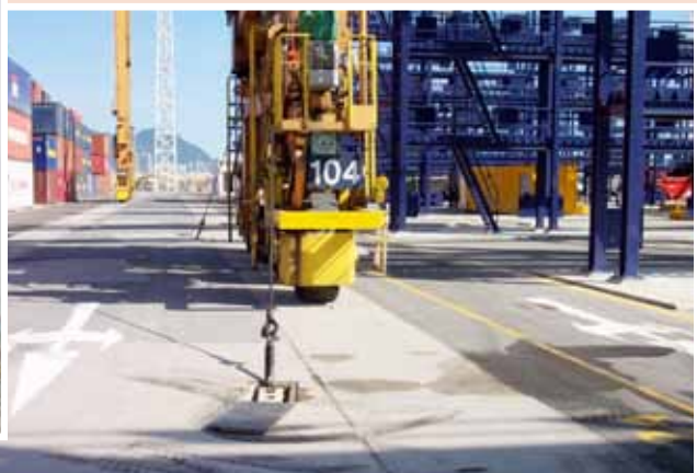
▲ Cranes anchored with steel wire (photo provided by HIT)
