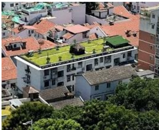
Green roofs in Wuhan, China
