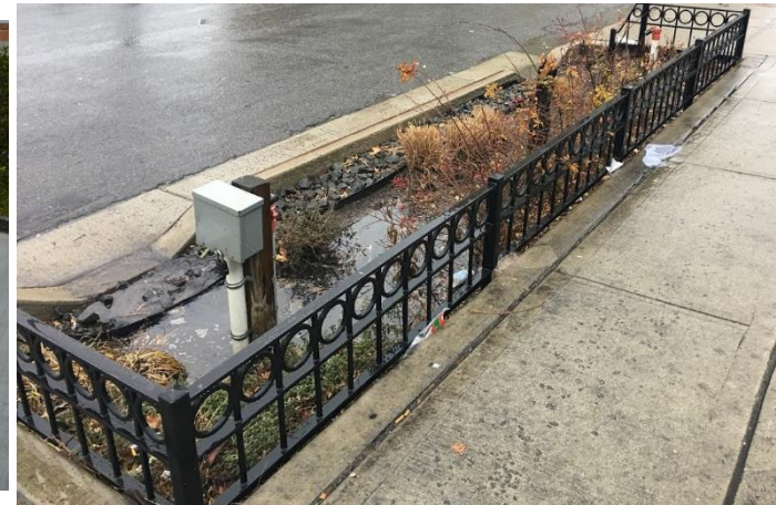
Right-of-way (ROW) bioswales in New York City
