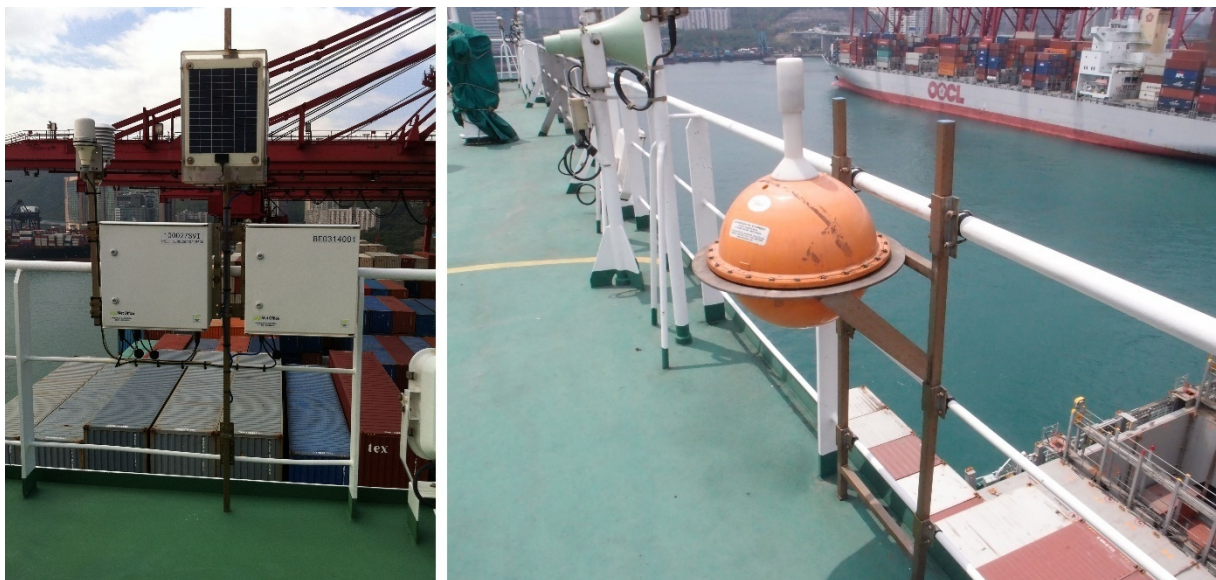
Figure 6 - Automatic weather station installed on board Hong Kong VOS, providing hourly measurement of atmospheric pressure and temperature over the seas.
