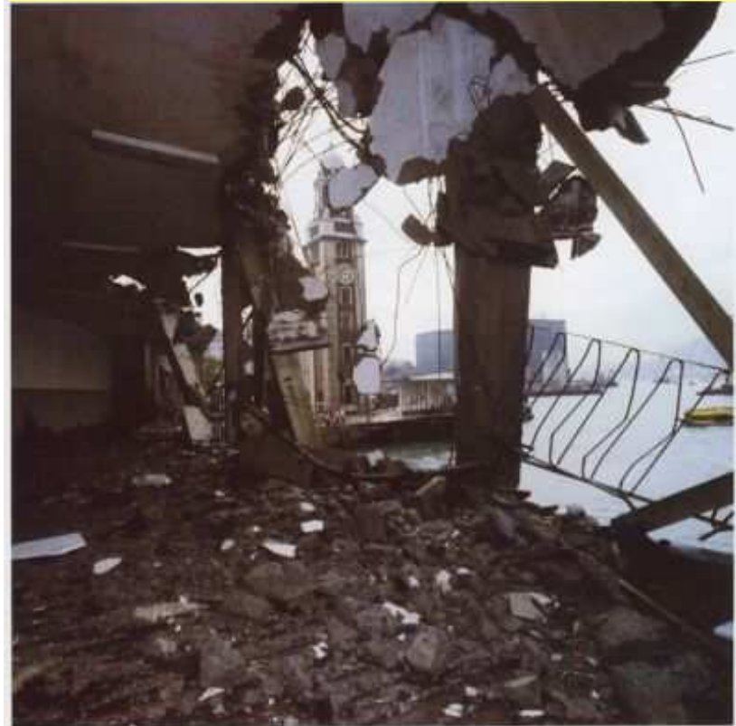
Fig. 2.27. View of the Tiou Shek Tin clock tower through the twisted rubble of Star Ferry Pier, which was damaged by a container ship during the passage of Typhoon Hobe (August 1979). Courtesy Hong Kong SAR Information Services Department.
