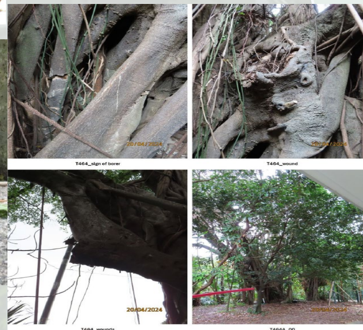
Tree inspection done a Ficus microcarpa
