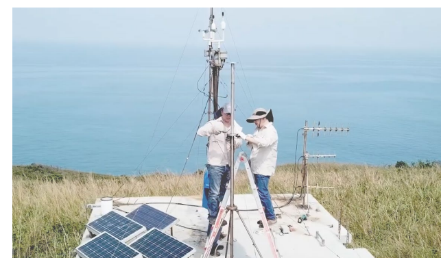
Equipment installation in outstation
