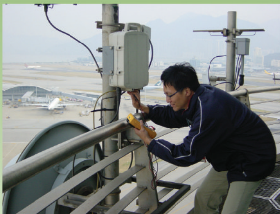
安裝設備後進行詳細測試 Carefully testing equipment after installation
